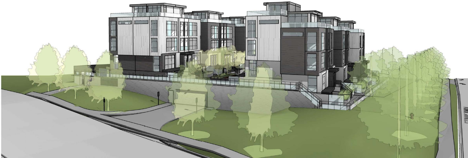
2 RIDGE ROAD VIEW
